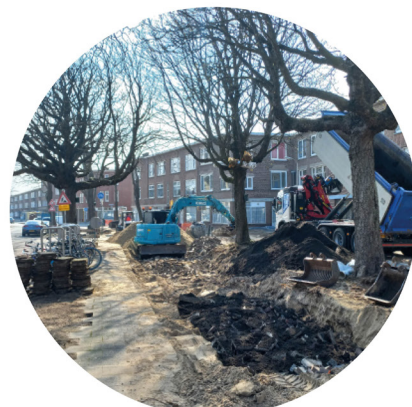
FIGURE 9 Design principle B: vital soil in constrained areas. Close attention is paid to all technical solutions that will make it possible to link the various open soil spaces. To improve the soil in more challenging sites, for example, due to paving conditions and/or car traffic, techniques known as 'second soil levels' can be used; these retain water under the paving and allow more oxygen to penetrate the soil.
