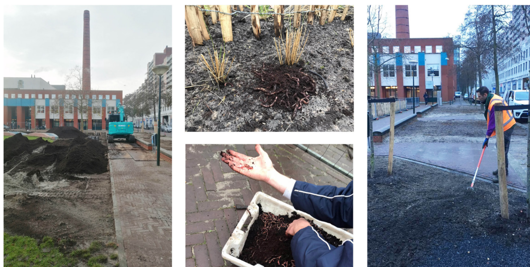
FIGURE 13 Pilot project 1: Park Slachthuisplein – soil development. A site-specific method to sustainably enrich the soil was defined. Instead of being replaced, the first 40 centimetres of the soil was mixed with specific compost, biochar, and worms. Soil profile rebuilding (Day & Bassuk, 1995; Heyman et al., 2019; Percival et al., 2023; Sax et al., 2017) was used to make the soil more fertile. A specific mix of compost, biochar, and earthworms was mixed through the first 40 centimetres of the soil (Darwin, 1882; Müller-Inkermann, 2020). The amount of compost was calculated to increase the percentage of organic matter from 1–2% to 4–5%. At locations with grass, the existing soil was somewhat more fertile than locations under pavement. These variations will result in slightly different microhabitats, microbiology, and plant species. A mulch layer did not fit into the budget, so we used litter and dead plant residues in the first autumn as a starter for a mulch/litter layer.
