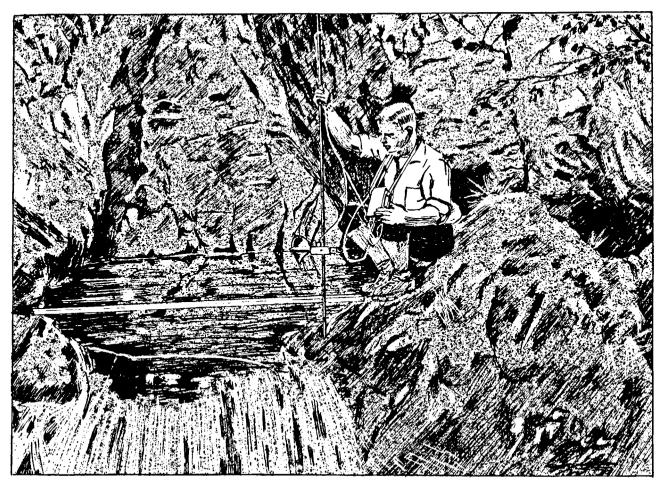
Fig. 11.4 Discharge measurement of the Pila-karst spring.
