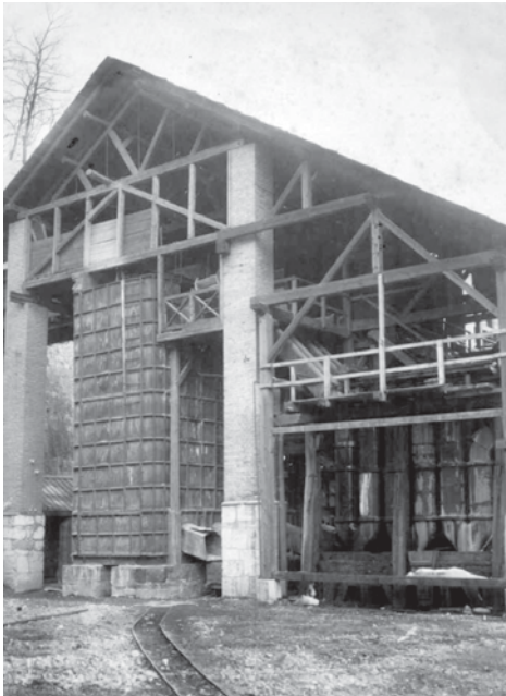
Fig. 3. Shaft furnace (Exeli system, 1872).
