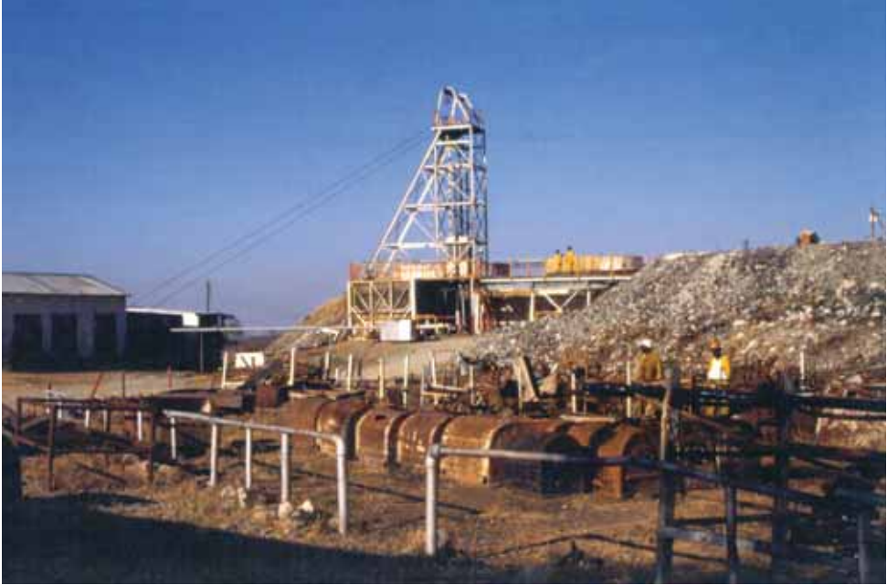
Fig. 25. The main production shaft at Zeus mine serving as haulage shaft down to 400 feet (122 m).
